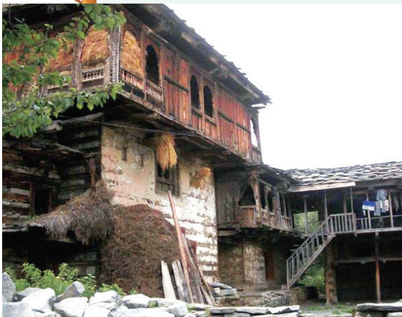
Fig. 1.6. Kath-kuni House, Himachal Pradesh
