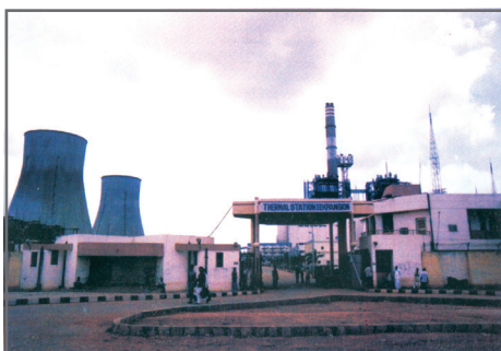
Fig 3.10: A view of a Thermal Power Station
